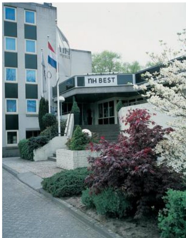
View of hotel facade
