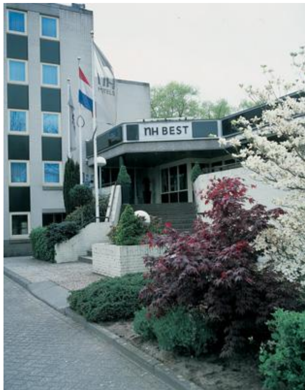
View of hotel facade
